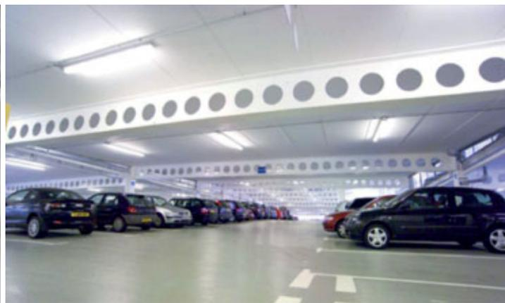
Fig. 2 - Internal views of steel framed open car park structures.
