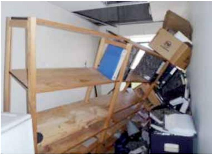
Fig. 2 - Collapsed ceilings and contents in a moment framed building
