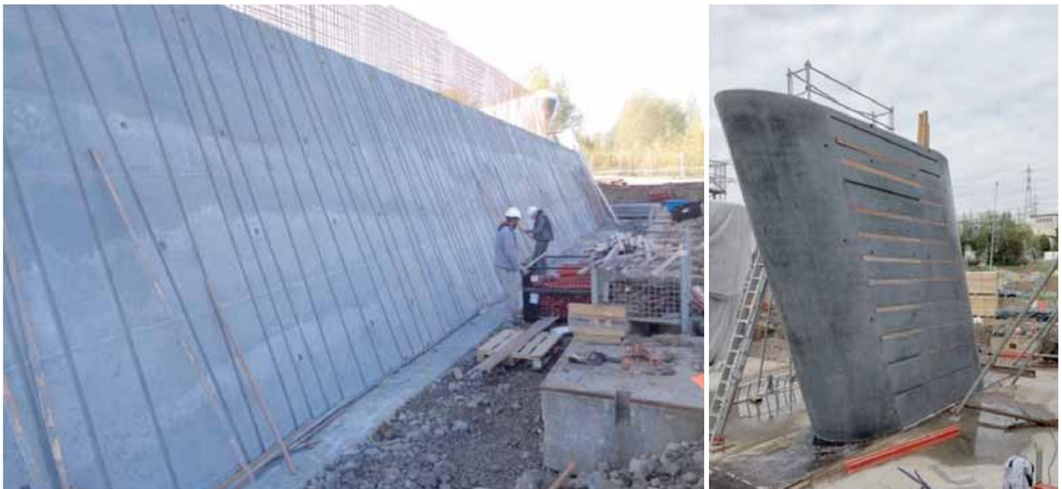
Fig. 5 - Abutments (left) and pier (right) under construction
