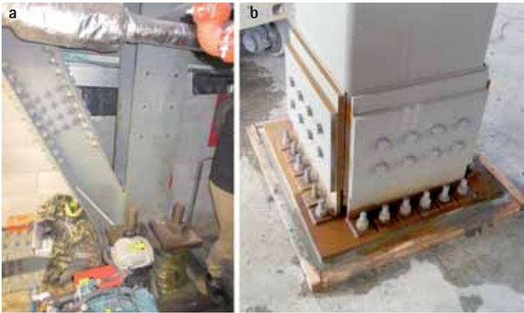
Fig. 5 - Examples of column bases that keep the column dependably elastic in a severe earthquake. (a) Spring Uplifting Column Base [C. Clifton]. (b) Sliding Hinge Joint 2 Way Acting Column Base [C Clifton]
