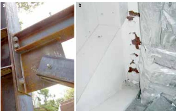
Fig. 7 - Beam/brace/column connections allowing for deformation capability. (a) Beam/brace/column connection designed for gap opening and closing. (b) Photo of beam/brace/column connection in EBF building, 21 February 2011 Christchurch earthquake
