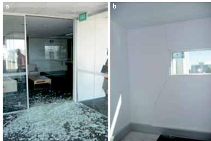
Fig. 4 - Effects of vertical acceleration on HSBC Tower. (a) Dislodged glass door [C Clifton] (b) Cracking to internal linings of window-box. [C Clifton]
