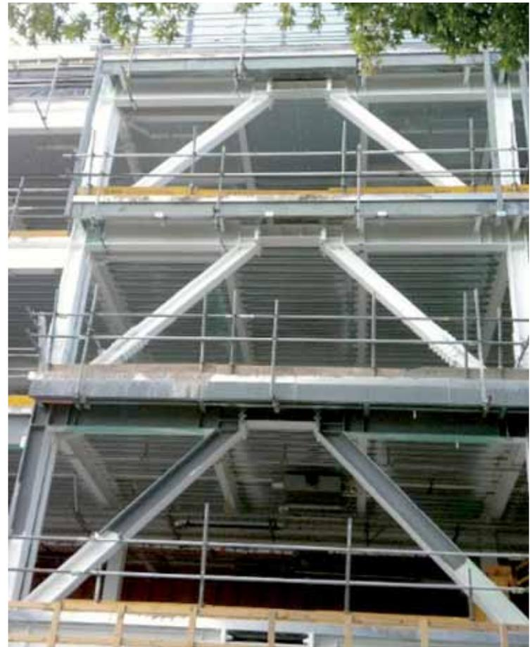
Fig. 10 - EBF with bolted replaceable active link from the rebuild of Christchurch [C Clifton]
