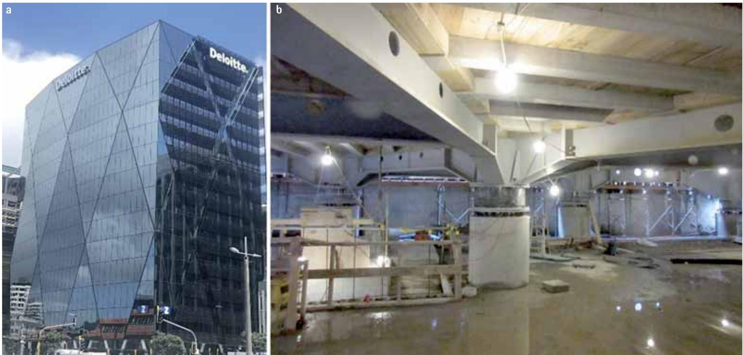
Fig. 13 - Base Isolated Office Building, Wellington, New Zealand. (a) External view of building [C Clifton]. (a)Base isolators underneath the ground floor [C Clifton]-
