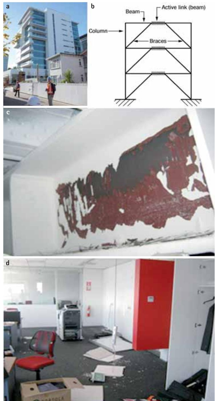
Fig. 1 - HSBC Tower following the 22nd February 2011 earthquake. (a) Overall view of tower from North West Corner [M Bruneau]. (b) Member terminology for a V braced EBF [NZS 3404]. (c) Inelastic demand in EBF active link [C Clifton]. (d) Typical interior of office following 22 Feb 2011 earthquake [C Clifton]
