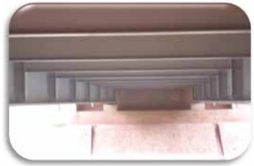
Fig. 6 | Cross beams and vertical stiffeners
