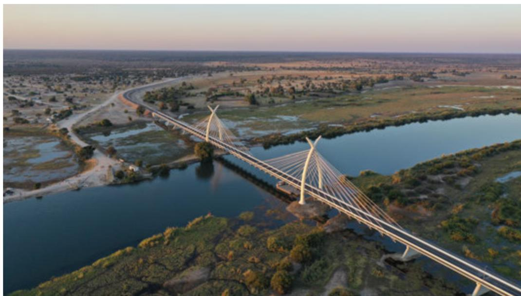
*of carriageway, supported by two main steel girders in double T section spaced by 6,2 m, with a constant height of 2 m, and a secondary girder along the bridge axis supported by the diaphragms.*
