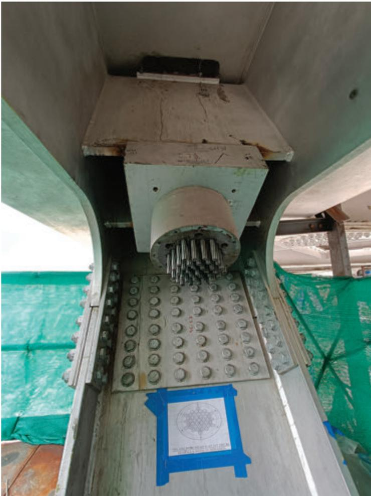
Fig. 10. | Anchorage dead end at deck side
