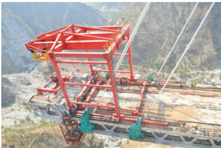
Fig. 18. | Gantry launching the first cantilevered deck segment (the No. 25)
