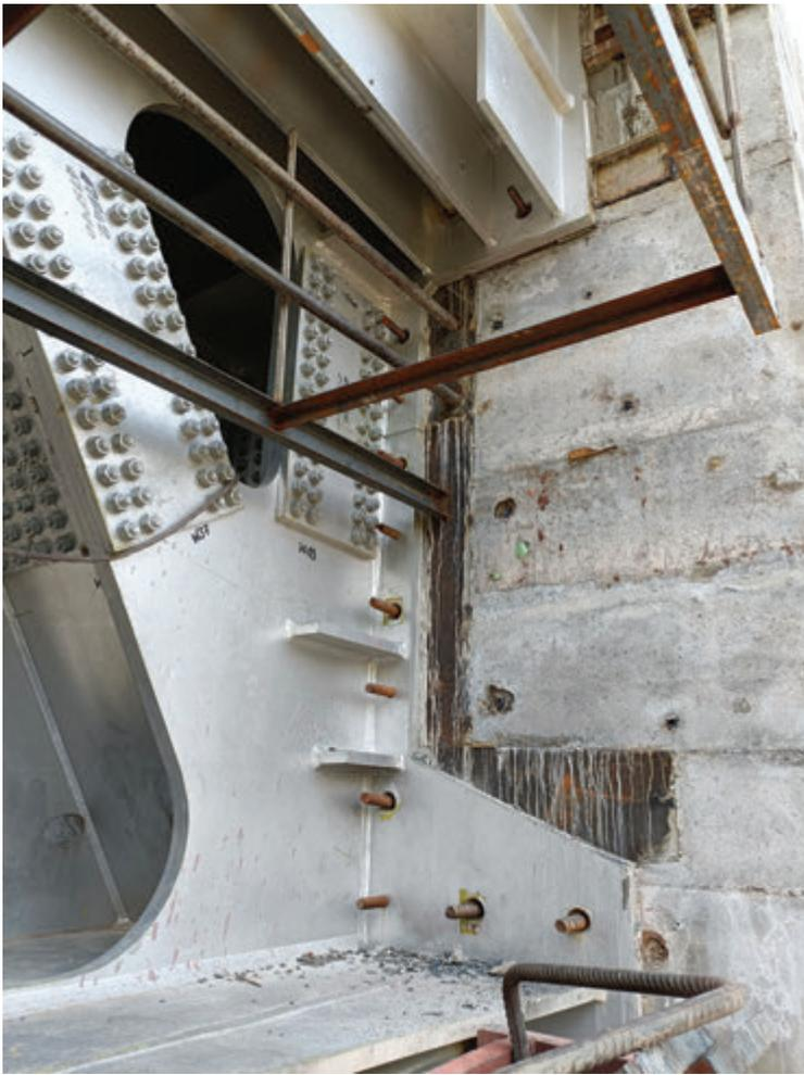
Fig. 14. | Truss beams structural connection with MA2 abutment
