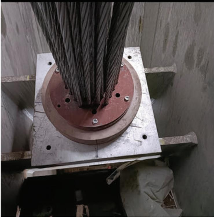
Fig. 9. | Anchorage stressing end at tower side
