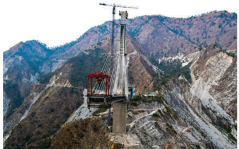
Fig. 19. | Cantilever construction of the main span, up to date
