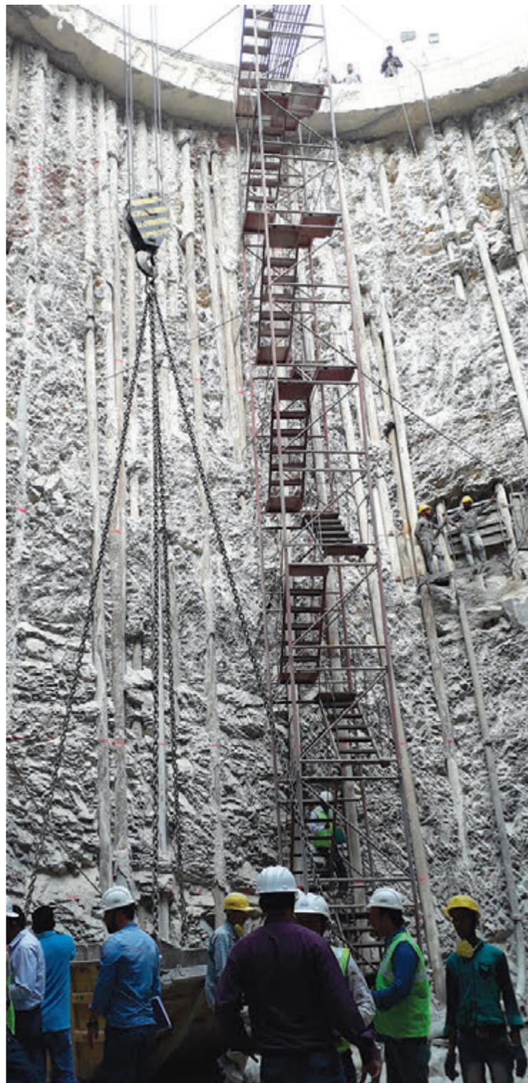
Fig. 3 | Tower well foundation during the excavation
