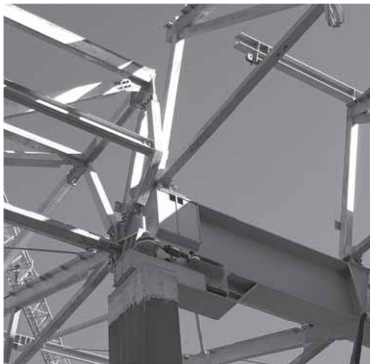
Fig. 9 | Nodo in opera con shock-transmitters
